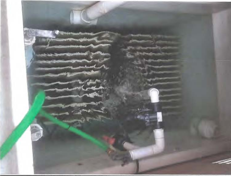
Filter grids replaced on the phase 1 rec pool
